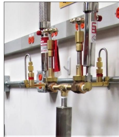
Picture 30 – Bronze Cryogenic Globe Valve
