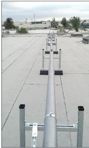
Picture 4 – Synthetic Roof Pipe Support
