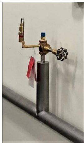
Picture 29 – Bronze Cryogenic Globe Valve
