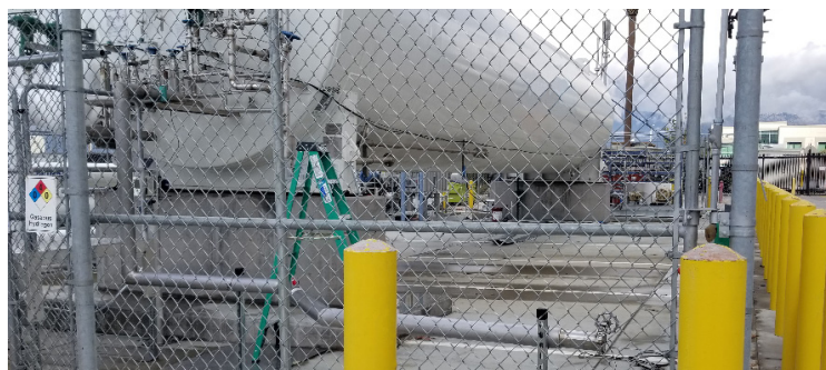
LH2 Vacuum Insulated Pipe and Extended Trailer Fill Lines
