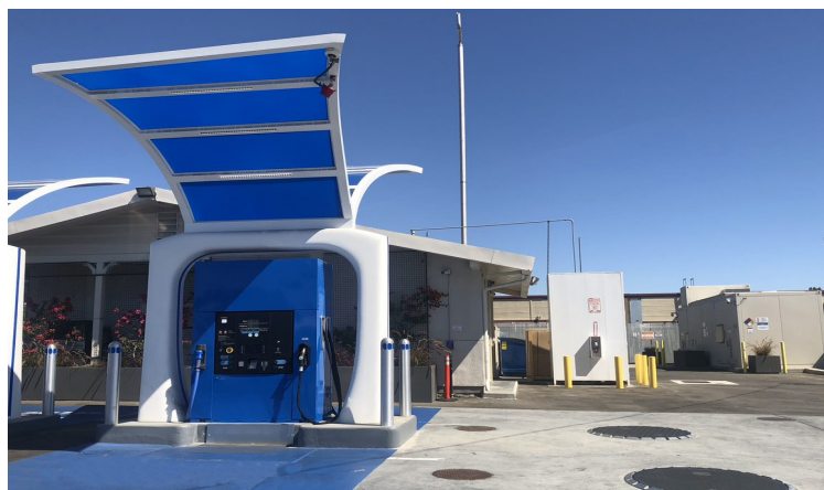
Hydrogen Fueling Station - Vacuum Insulated Lines
