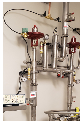
Automatic Dewar Switching Manifold
