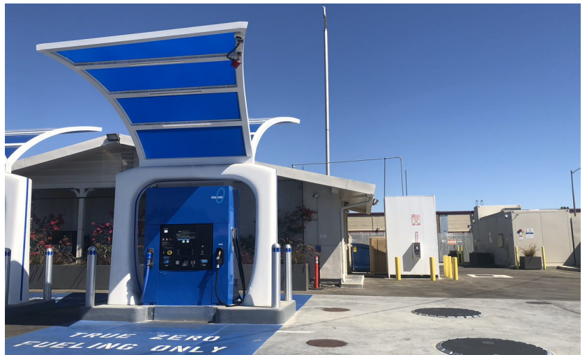
Hydrogen Fueling Station - Vacuum Insulated Cooling Lines
