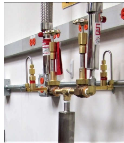
Picture 26 – Bronze Cryogenic Globe Valve
